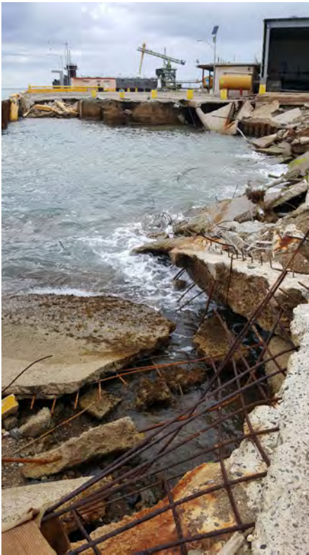
Damage at the port in Mayaguez
