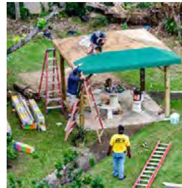
Delivery drivers for FEMA contractor Estes Express Lines volunteer at the Hogar Escuela Sor María Rafaela school for girls in Bayamon on February 1, 2018. The volunteers repaired damaged roofs, tables, benches, and playground equipment during their free time.
